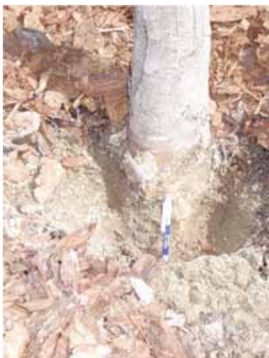
Fig. 2 Excavating around the base of the trees
